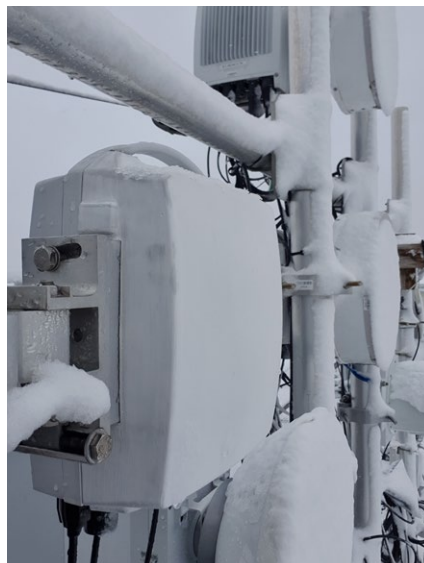
Antenna with water-repellent coated radome
