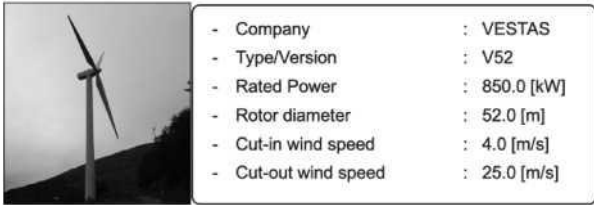
Figure 4. Windmill specifications
